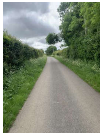
Photograph 22: Existing Conditions along Lomer Lane
