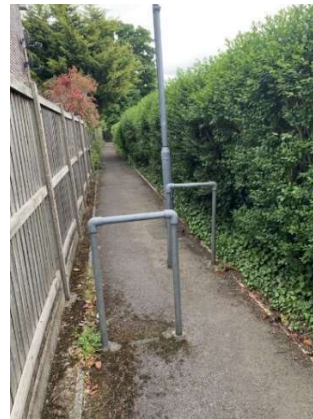
Photograph 8: Footpath at Route 'I' Ringwood Road End
