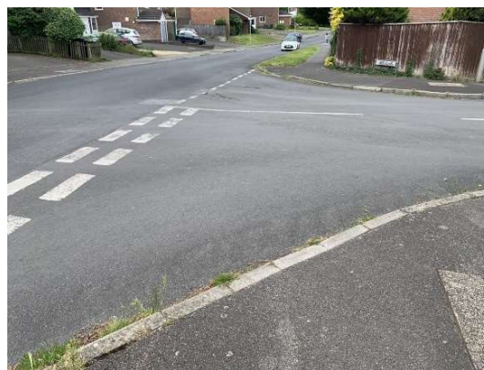
Photograph 18: Pedestrian Infrastructure along Earlswood Drive
