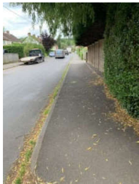
Photograph 3: Footway along Ringwood Road
